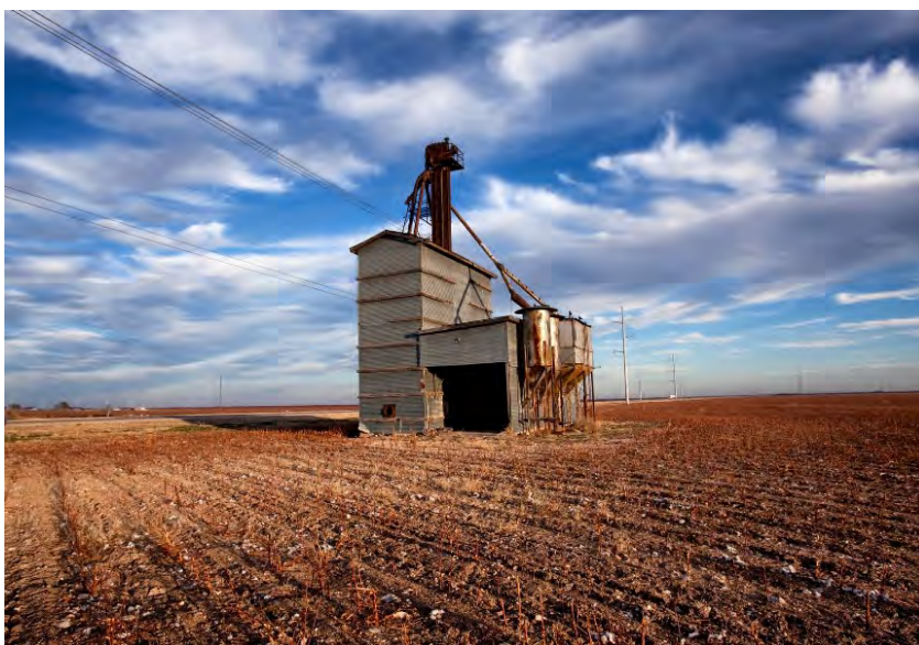
Figure 11. Abandoned grain elevator in ghost town of Wastella, Texas
