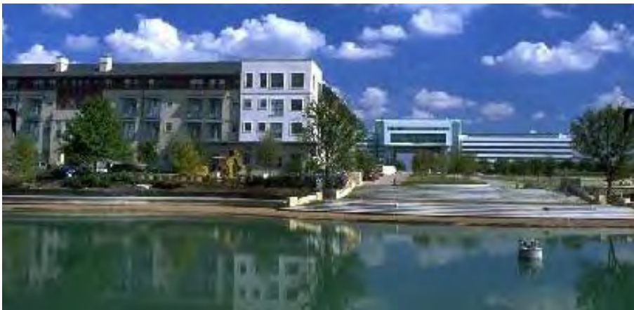
Figure 68. Legacy Town Center in Plano, Texas – a Good Example of Mixed Land Uses, One of the Ten Smart Growth Principles
